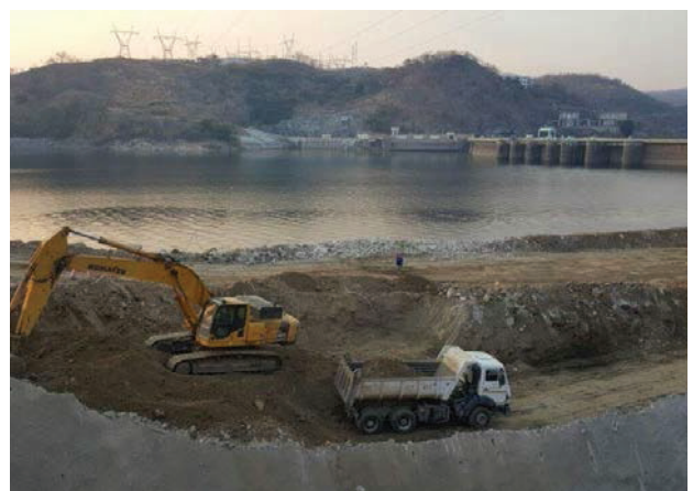
Kariba South Power Station Expansion Project
