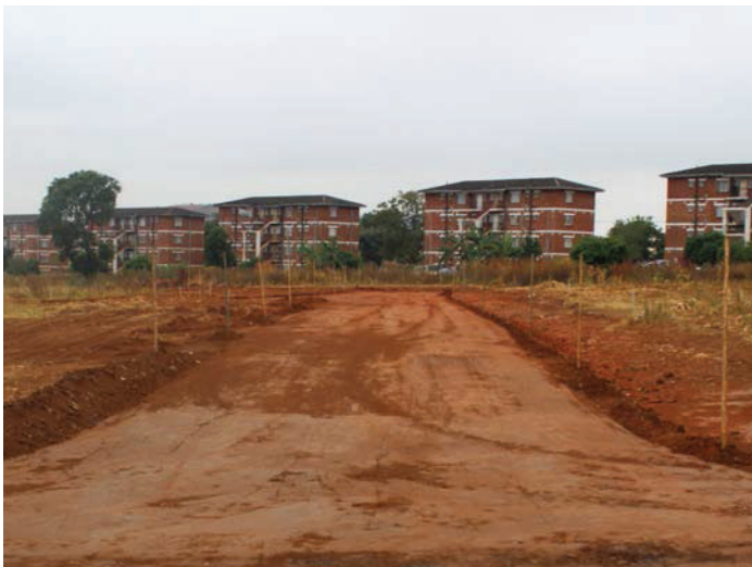
New Marimba Park (servicing in progress)
