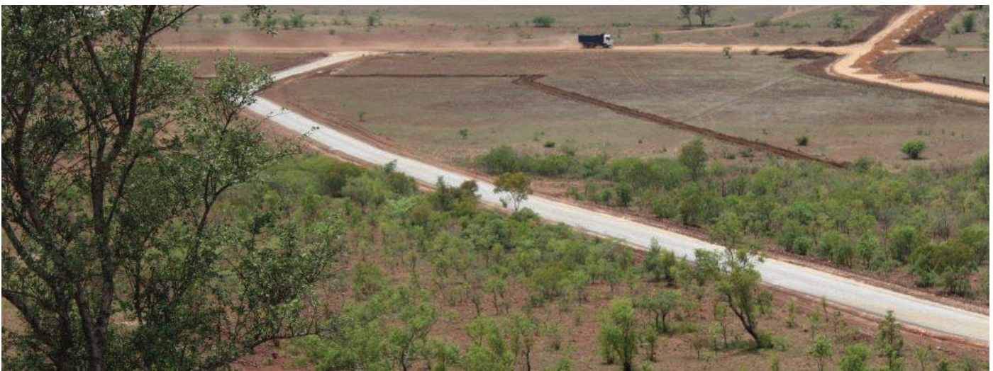
Servicing in progress at Clipsham Views Housing Project
