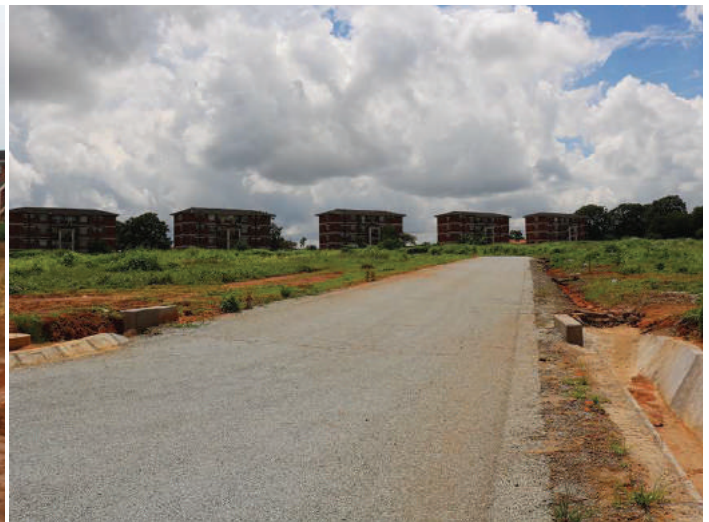
New Marimba Park (servicing completed)
